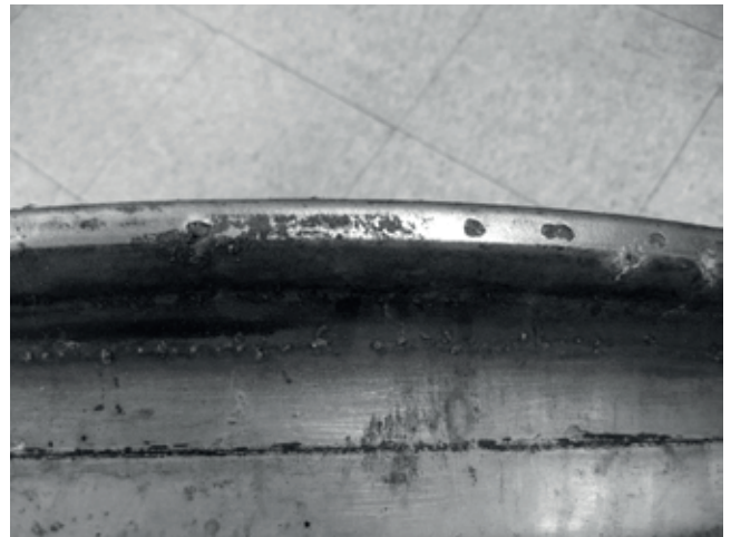
Picture 13-38 Acceptable pitting
